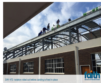
DAY 472: Isolation rolled out before cladding is fixed in place
