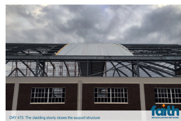
DAY 475: The cladding slowly closes the support structure
